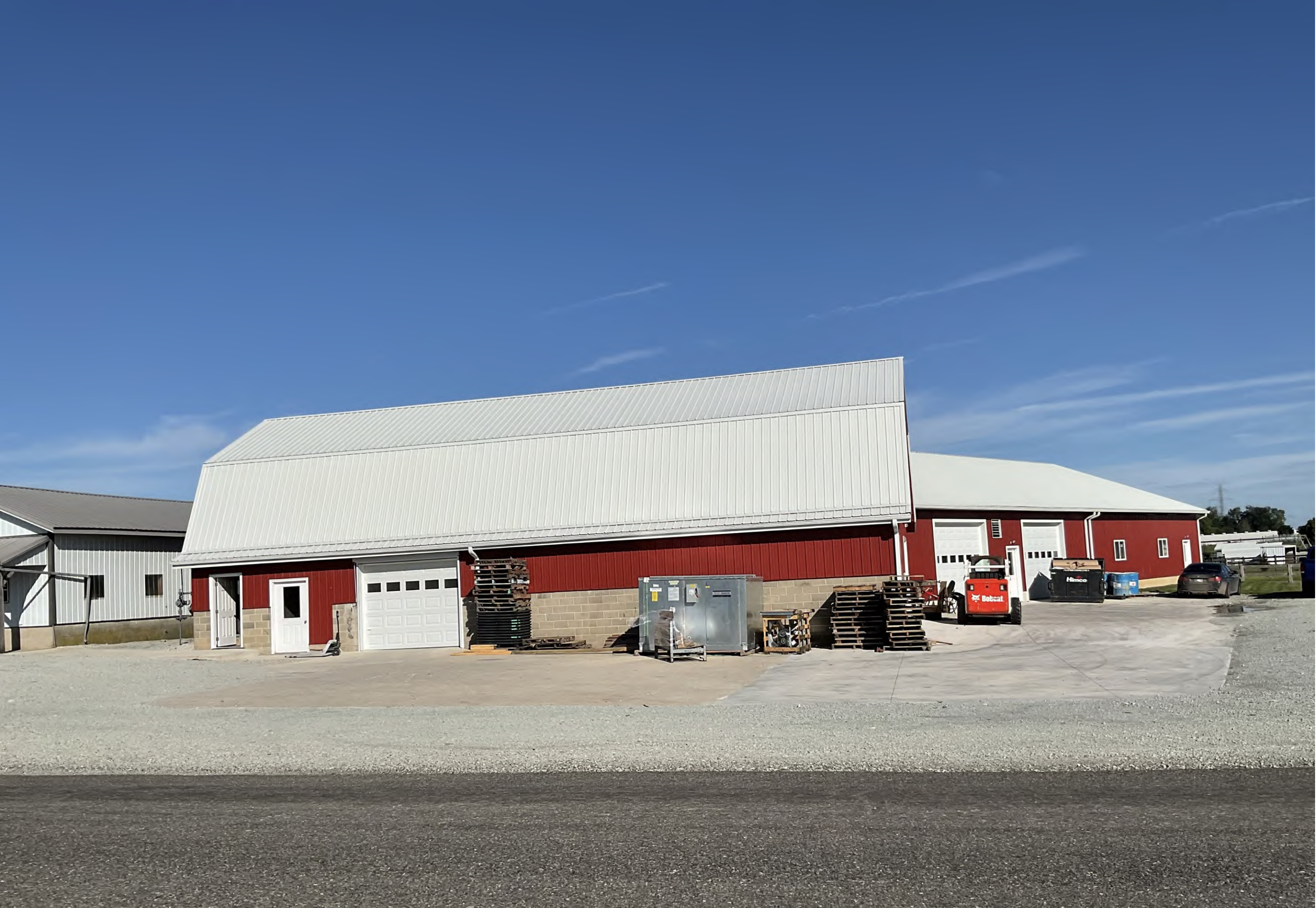
Subject property existing workshops
