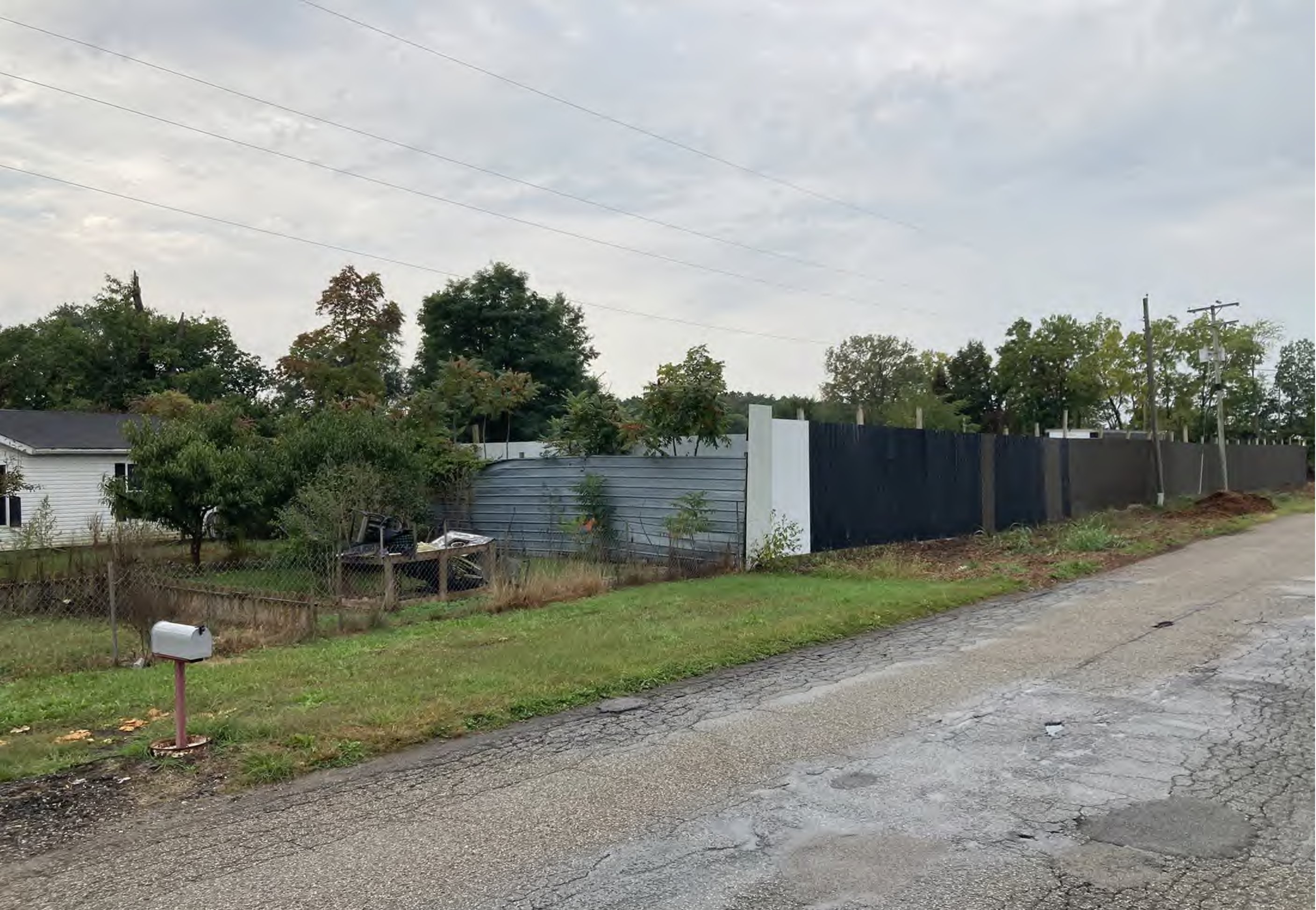
Subject property (northeast corner)
