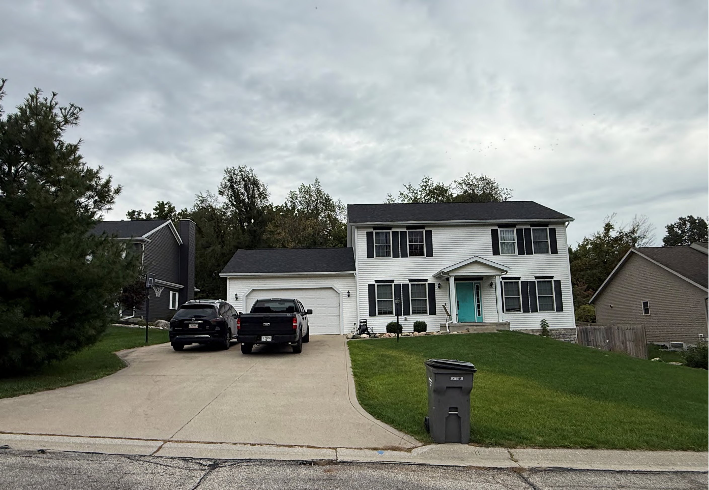
Subject property facing east
